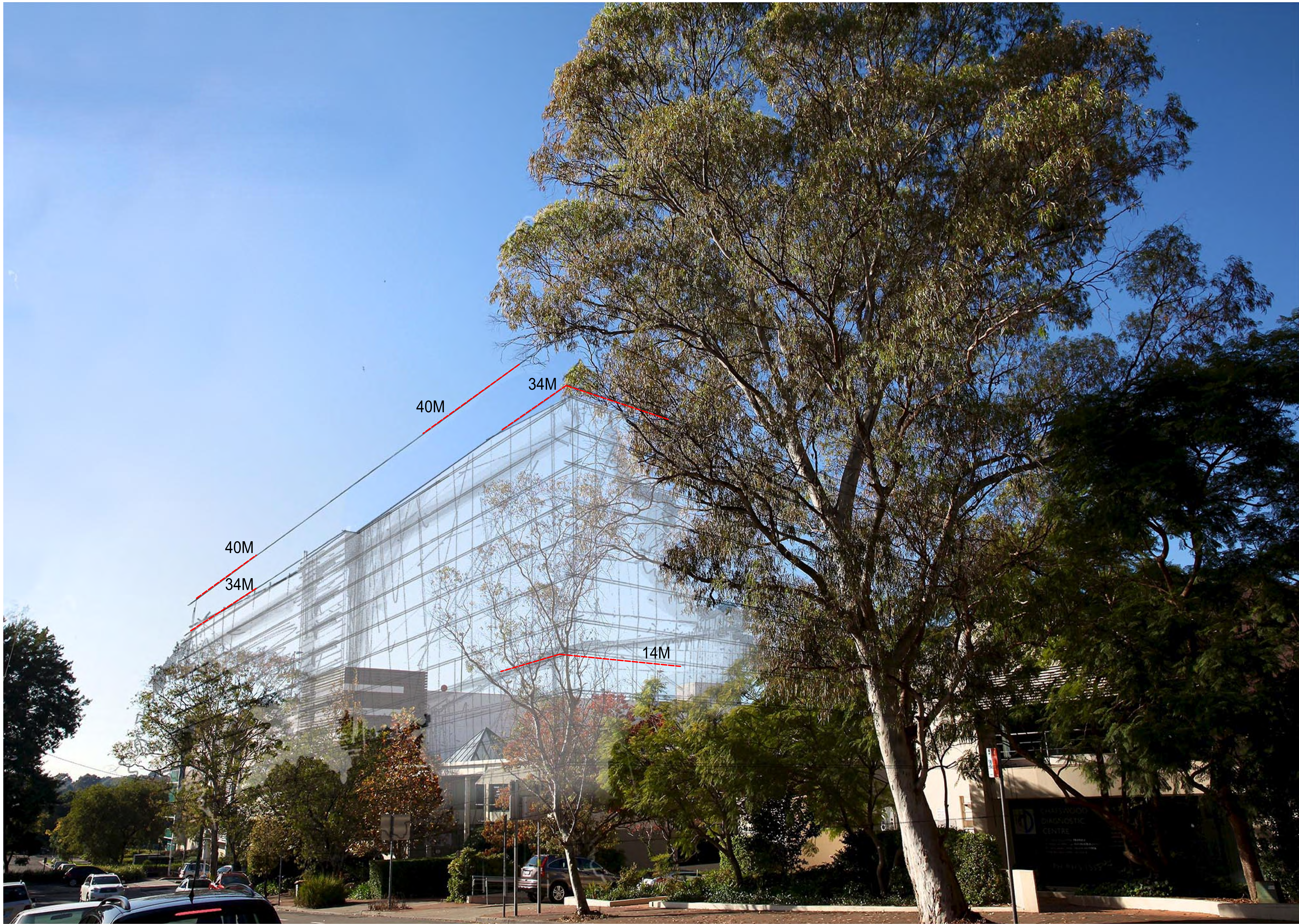
VIEW 2 MALVERN AVENUE LOOKING SOUTH EAST
